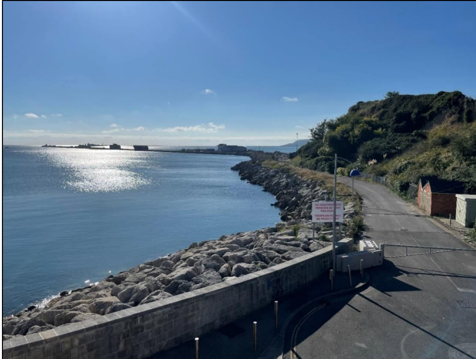
Figure 1 – Photo of entrance into site with existing retaining wall
